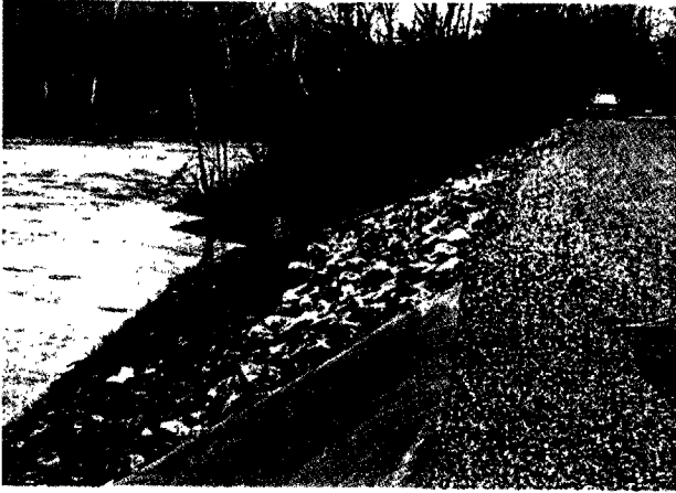
Photograph 23: Rip Rap at Edge of Parking Area Downstream from Draft Tube Discharge
