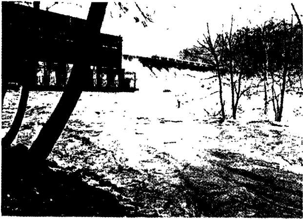
Photograph 5: Flood Level on Downstream Side of Powerhouse
