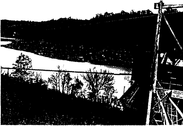
Photograph 1: Overview of Dam Facilities and Reservoir During Flood
