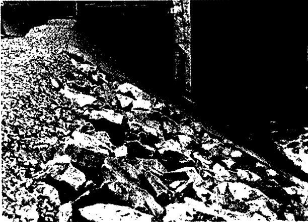
Photograph 22: Concrete Revetment and Rip Ram Adjacent to Draft Tube Discharge
