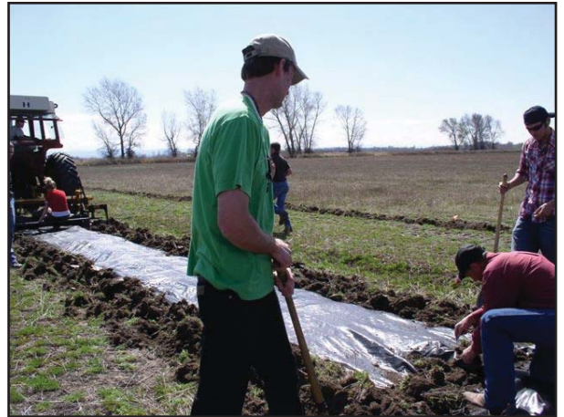
Volunteers lay weed barrier down to prevent weeds from growing around the trees and shrubs on the wetland.
