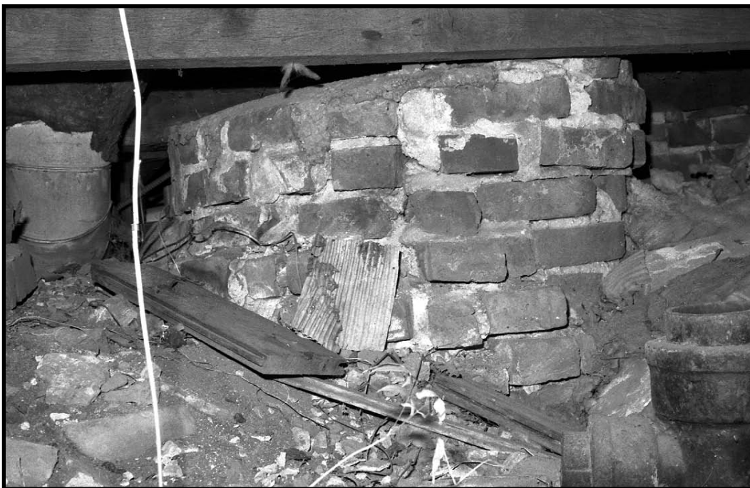
Figure 18. Cistern in Harriet Dean House crawl space.
