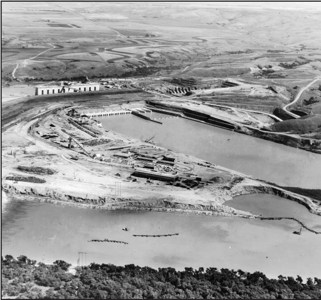
Fort Randall Dam under construction on the Missouri River in South Dakota. This was one of five massive dams constructed along the Missouri by the U.S. Army Corps of Engineers in the 1940s through the 1960s (RBS photograph 39CH00-59).
