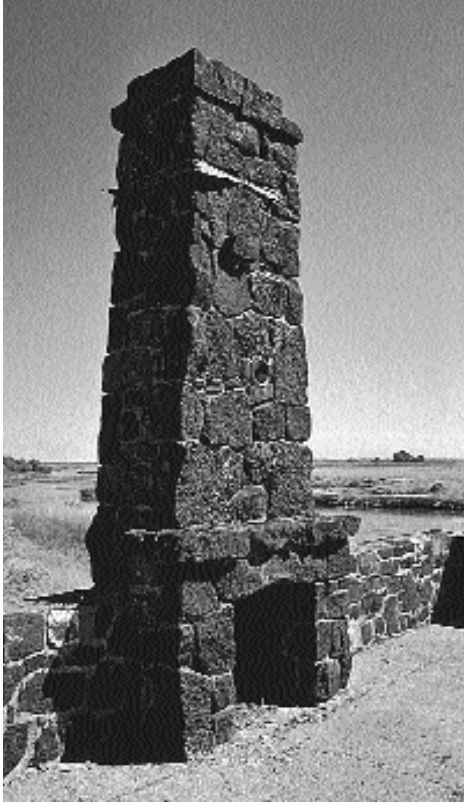
Chimney in waiting room of entry building. Photo by Dick Lord.
