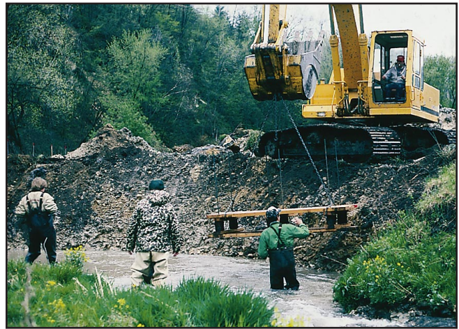
Trout habitat structures are installed to create fish habitat.
