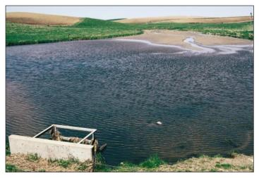
When watershed dams fill with sediment (above), the recreation, gully control, flood control, fish and wildlife benefits, emergency fire protection, road stability and many other benefits are lost. Other problems with aging dams are spillway breakup, deteriorating concrete, eroded berms, seepage through dams, cattle damage, and sloughing of dams.
