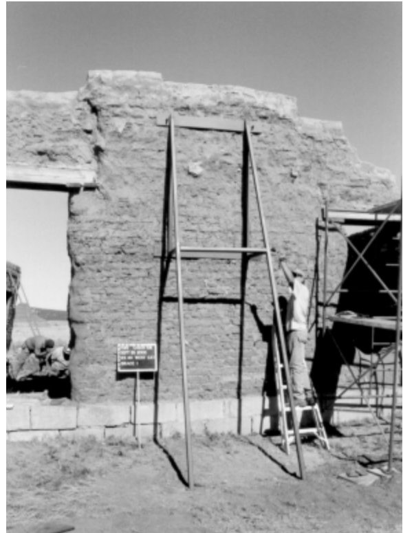
Bracing a historic adobe wall, Fort Union National Monument, NM.
