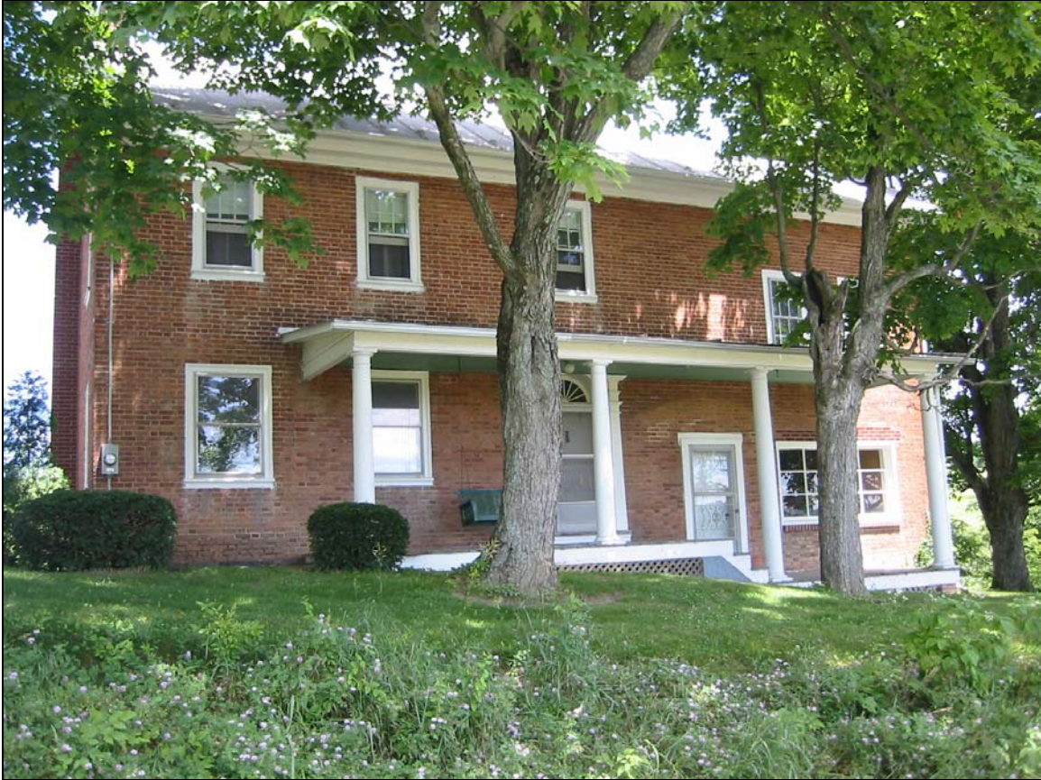
037-GR-003-02 House facade, looking NE. Alterations have cut off the Federal style fanlight, but the six over six windows on the upper story and the architectural detailing of the doorway suggest a date before 1840. Columbia County, Greenwood Township.
