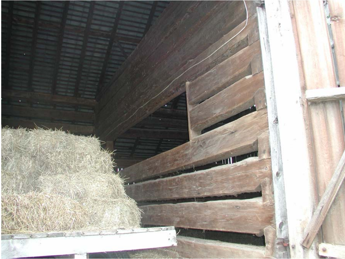
Dunlop barn, Potter Township (Georges Valley), Centre County, c. 1800. Above, east gable end showing Sweitzer profile; this photo, interior showing log crib and threshing floor.
