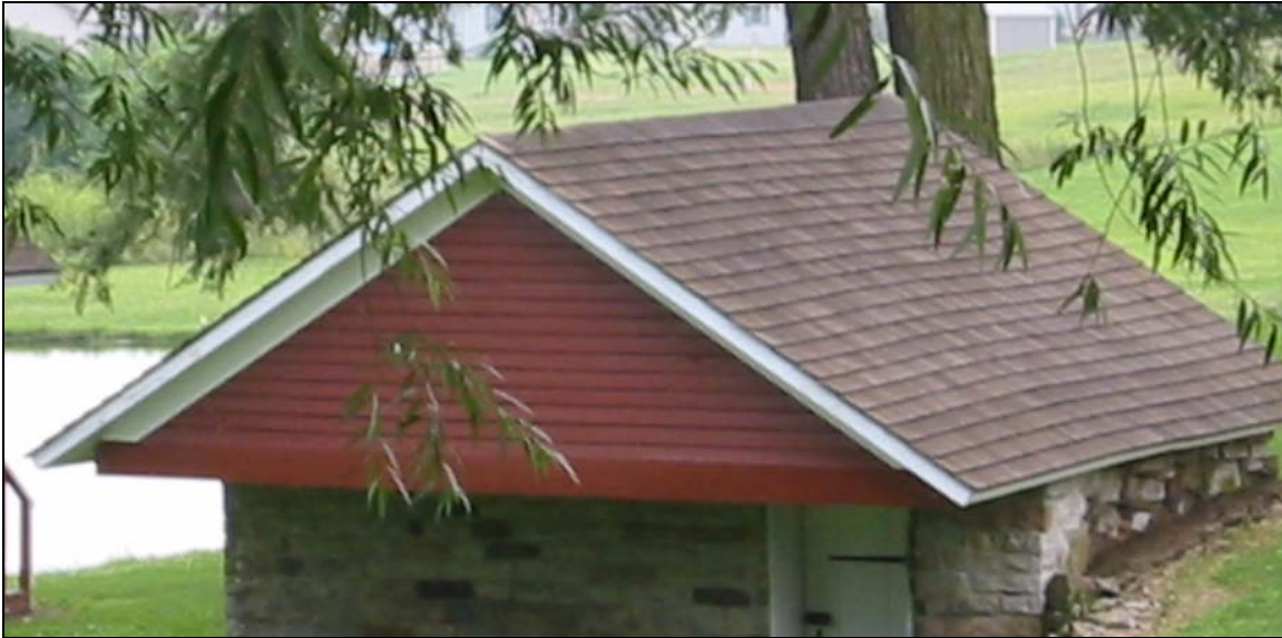
081-WO-001-03. Lycoming County, Wolf Township. The stone masonry, overhanging roof, and door hardware suggest an early 19 th century date. Note the telltale willow tree in the background.
