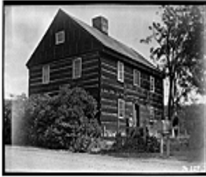
Center Chimney log cabin 24 in Terrytown, Bradford County, c 1806. Historic American Building Survey: Stanley Jones, Photographer September 1, 1936 SOUTH WEST VIEW OF EXTERIOR.HABS PA,8-TERTO,1-3
