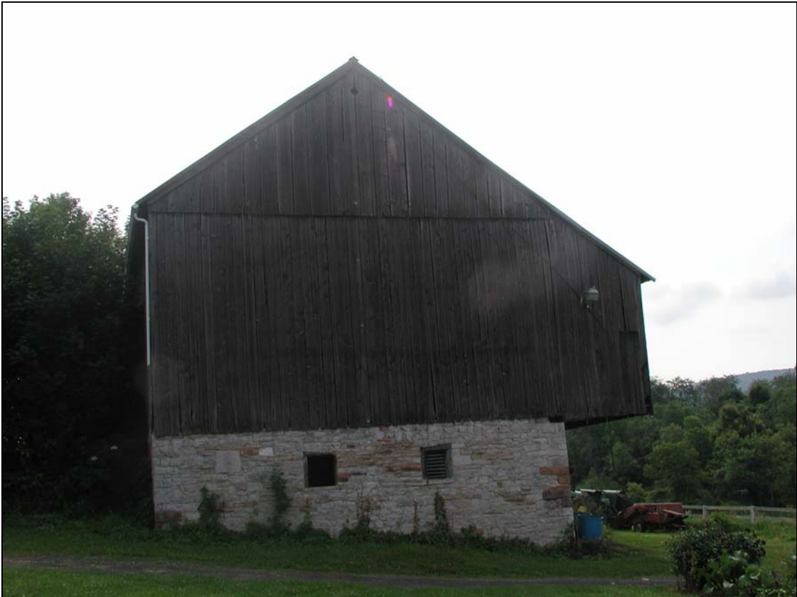
Dunlop barn, east gable end
