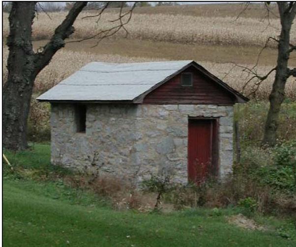
Spring house, Orndorf Road, Centre County
