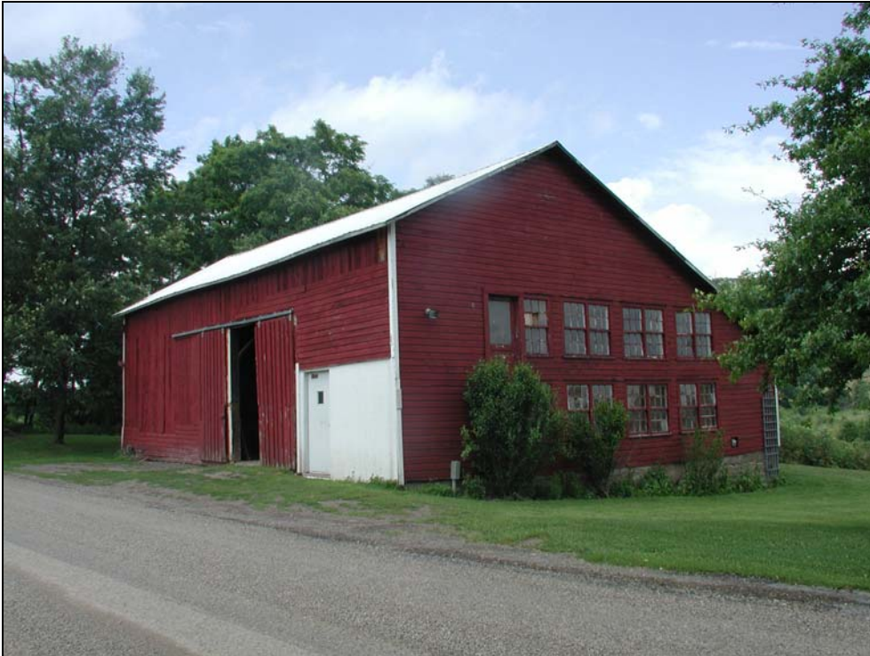
117-SU-003-02 barn from WEST 2. Tioga County, Sullivan Township. Three-bay English barn, c 1840-1850 (based on interior framing), with later alterations for poultry.
