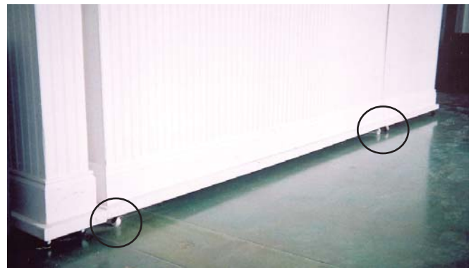
Detail. Casters on the bottom of the cubicle partitions allow them to be moved around or removed from the space.
