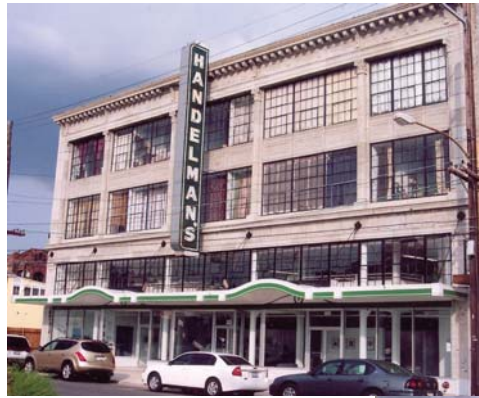
Left: This three-story building (shown after rehabilitation) was constructed in 1923 for use as a department store.
