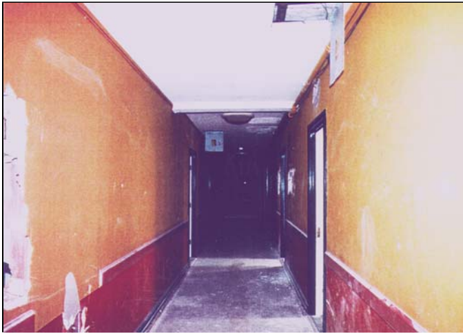
LEFT: Pre-rehabilitation view of typical corridor showing historic trim and deteriorated flat plaster.
