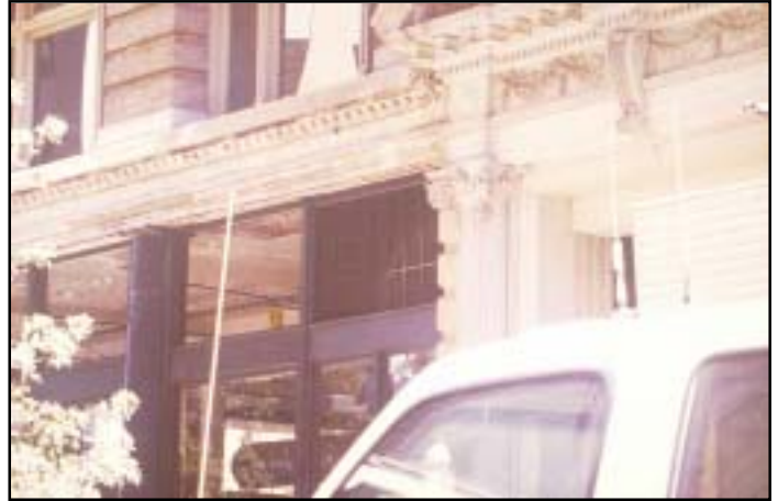
Detail of transom (under construction).
