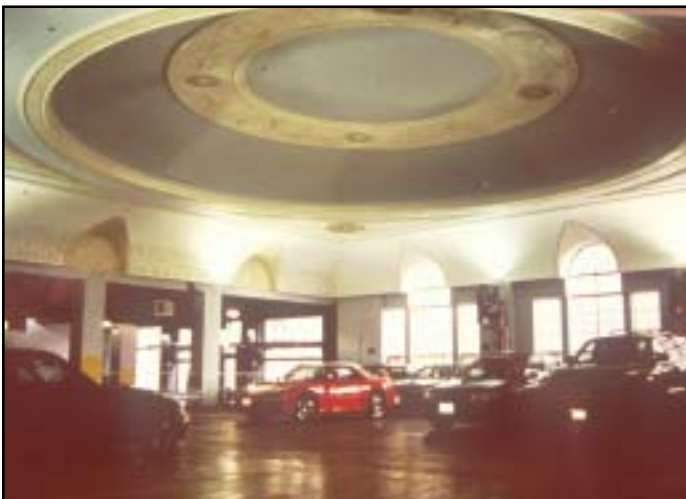
Parking cars in this highly-finished space is not a compatible treatment.
