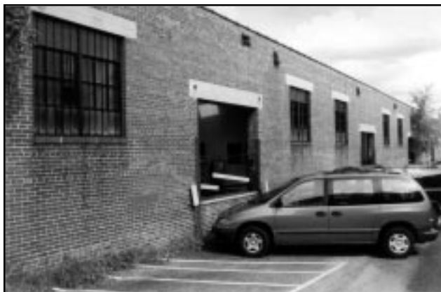
Loading door elevation after rehabilitation.
