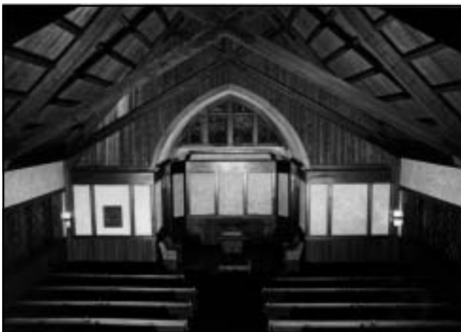
Sanctuary and apse before rehabilitation.
