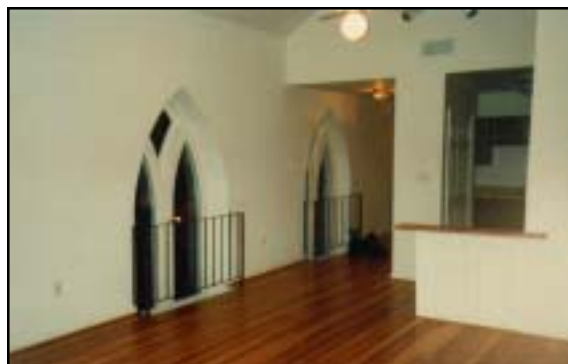
Sanctuary after rehabilitation with new floor and newly divided windows.
