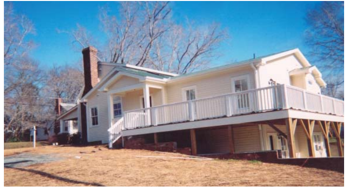
The size of this new rear addition—incorporating two floors and an extended depth—combined with substantial changes to the site overwhelm the modest historic house.
