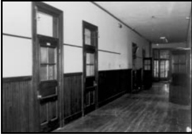
Second floor hallway prior to rehabilitation.
