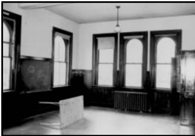
Second floor cloakroom, prior to rehabilitation.
