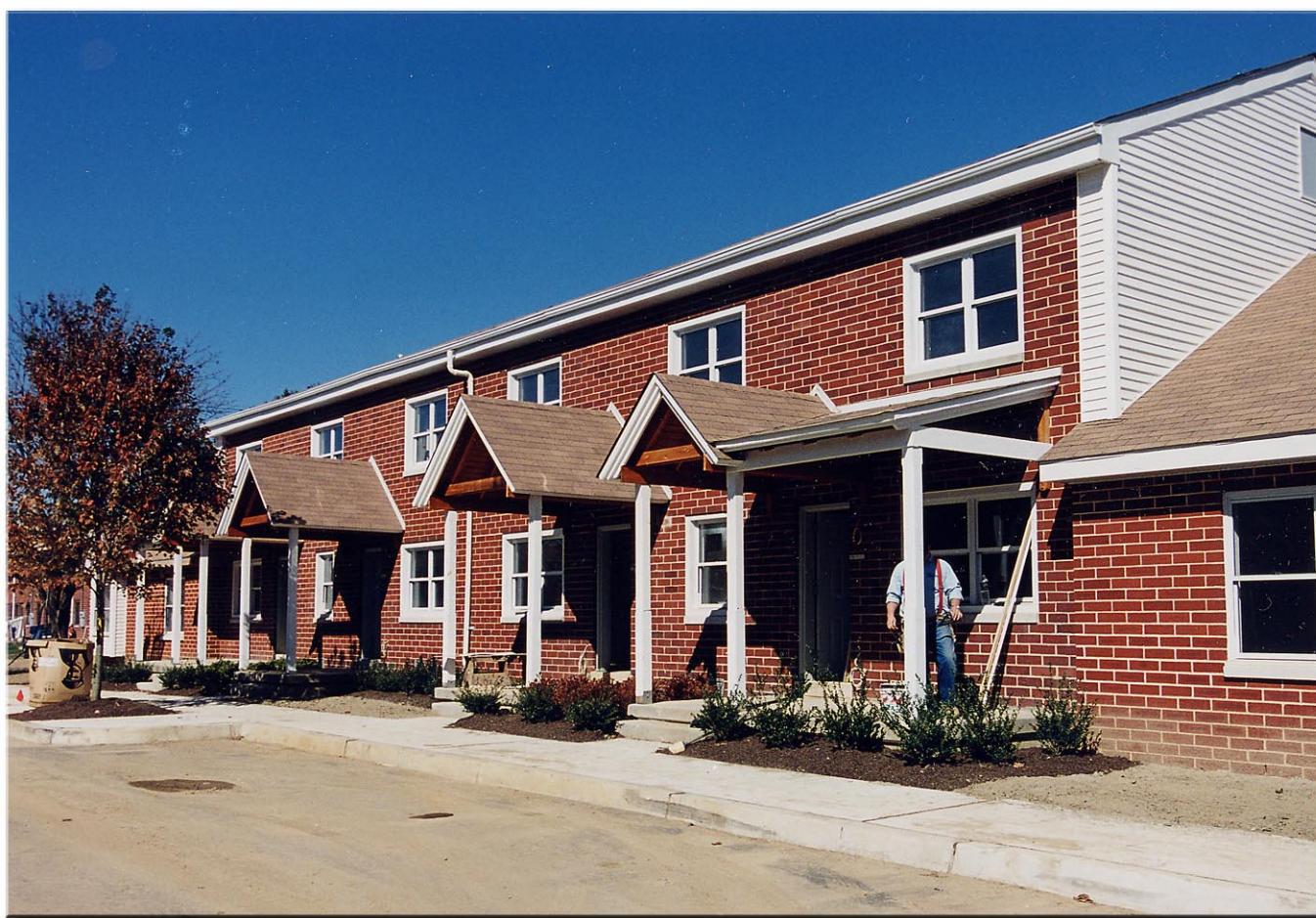
Camden Housing Authority, rehabilitated public housing development
