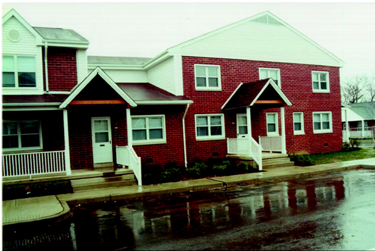
Camden Housing Authority, completed modernization project
