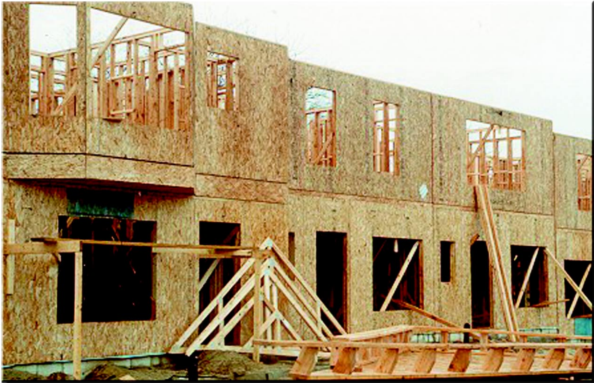
Camden Housing Authority, modernization project in progress
