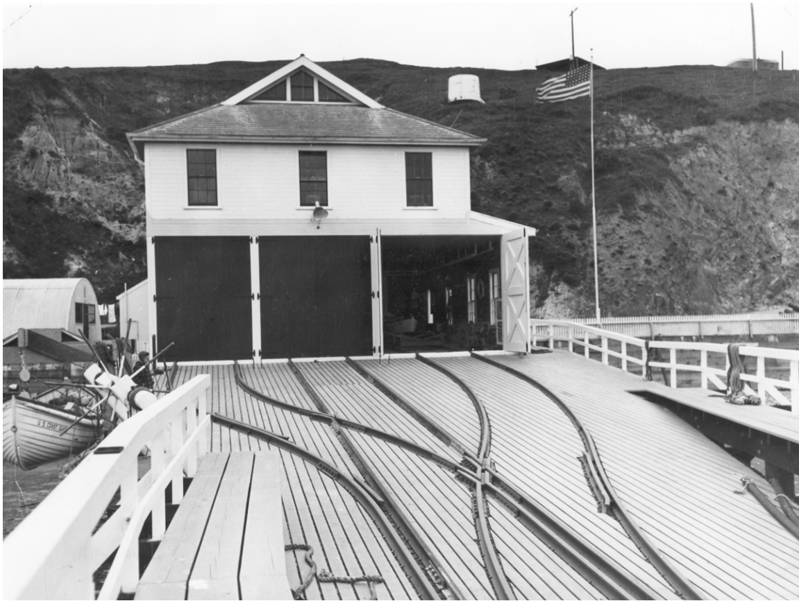
Photo #3 Point Reyes Lifeboat Station, Point Reyes, California. Front of the boathouse, showing the rail arrangement of the launchway, 1950. Courtesy of National Park Service.
