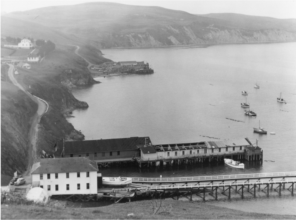
Photo #1 Point Reyes Lifeboat Station, Point Reyes, California. View of the station, looking E-S-E. Note the 36-foot lifeboat on the launchway, circa 1960. Courtesy of National Park Service.
