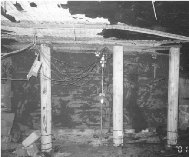
Figure 3. Photo of the replacement stopping at 33 crosscut
