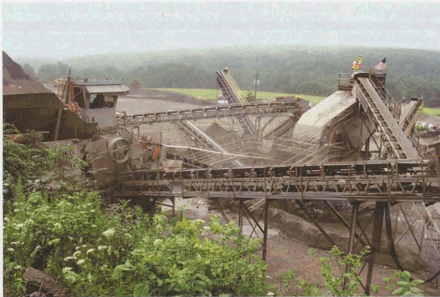
Surface crushing and sizing facilities.
