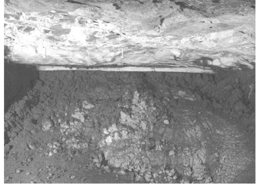
Figure 7. View of completed mine seal.
