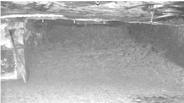
Figure 12. Underground view of mine seal No. 3-A from the B-Drift.
