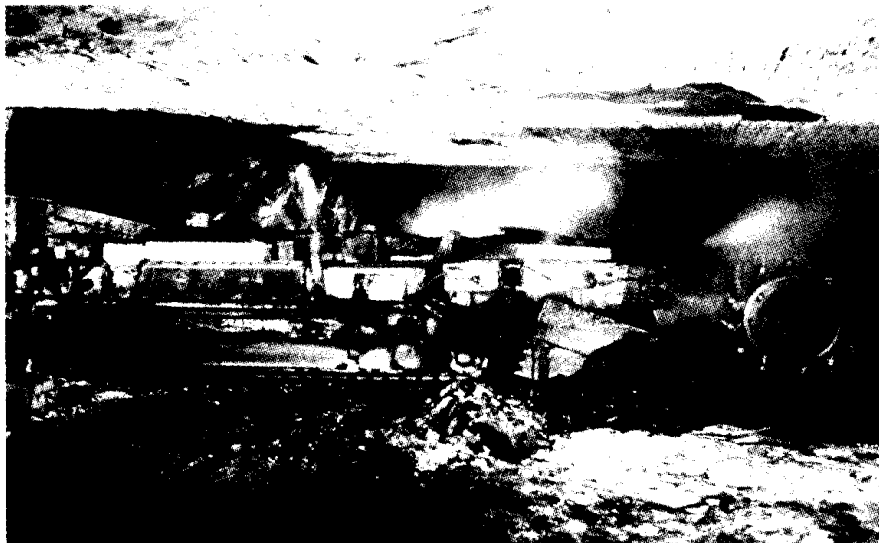
Fig. 26-1. Continuous miner. (From U.S. Bureau of Mines.)
