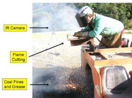
FIGURE 7. MINE WORKER PERFORMING FLAME CUTTING OPERATION
