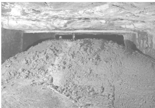
Figure 9. View of bulk fill placement for seal No. 2.
