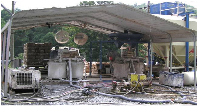
Figure 18. The two-components (powders) used to produce the CSA grouts are packaged separately in bags and delivered to the pumping site where they are mixed with water.
