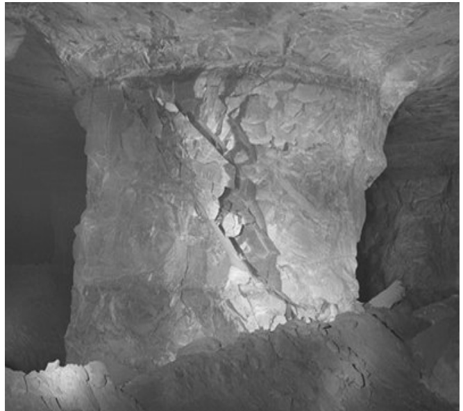
Figure 4. Partially benched pillar that failed along two angular discontinuities. Width-to-height ratio is 0.58 based on full benching height. The average pillar stress was about 4% of the UCS.
