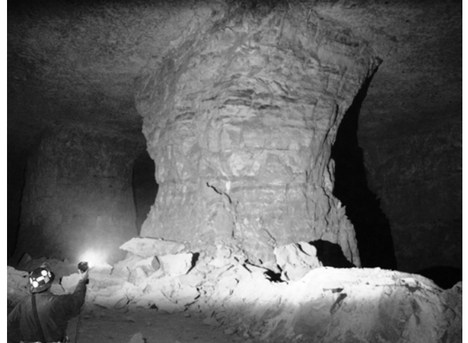
Figure 3. Partially benched pillar failing under elevated stresses at the edge of bench mining. Typical hourglass formation indicating overloaded pillar. Width-to-height ratio is 0.44 based on full benching height. The average pillar stress was about 12% of the UCS.
