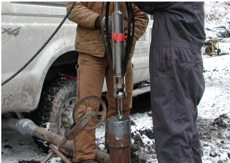
Figure 10. Remote video camera probe inserted into borehole near remote seal installation.
