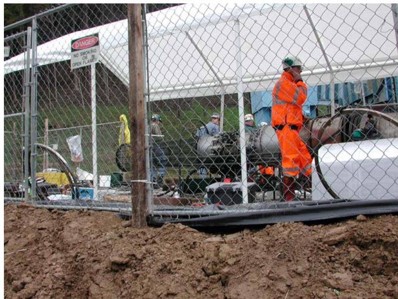
Figure 3. GAG engine installation.
