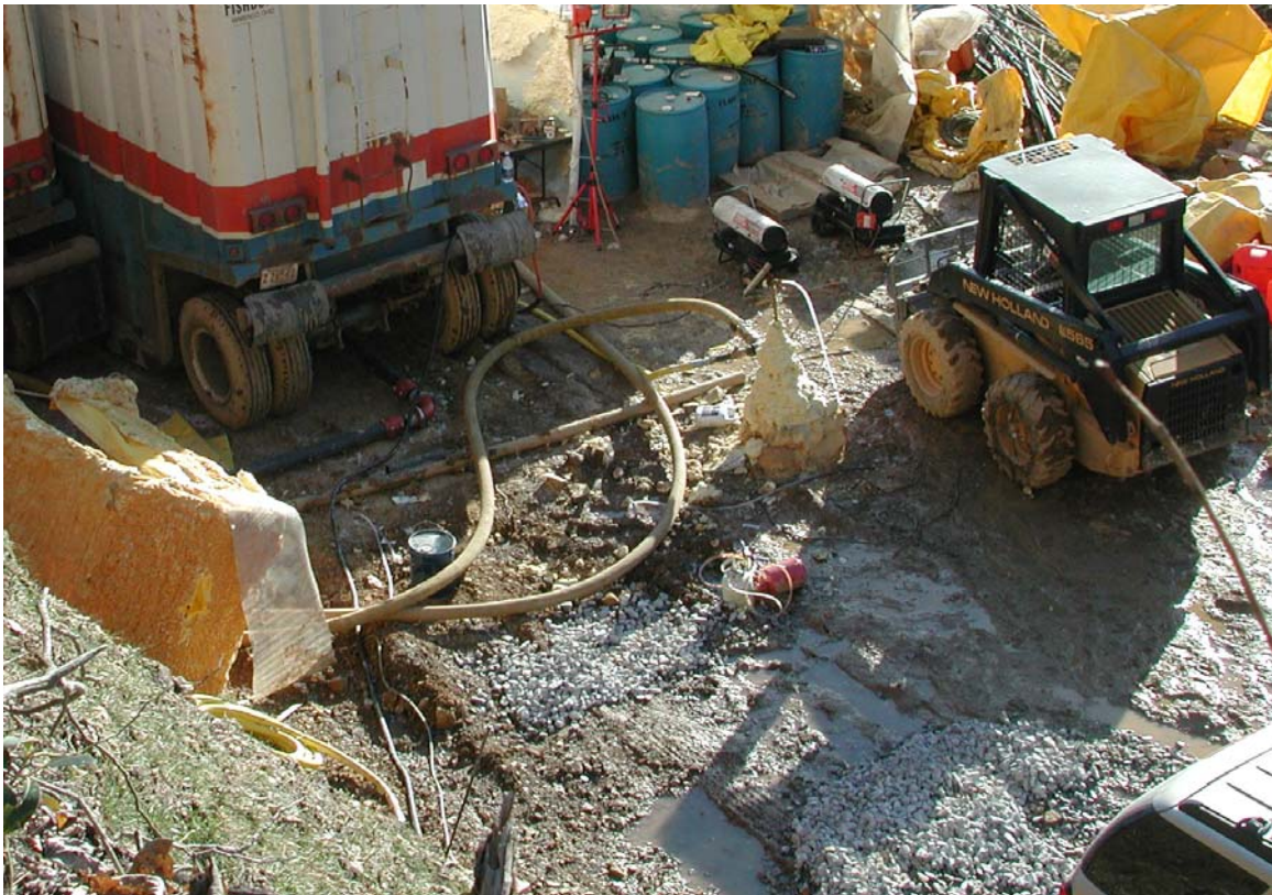
Figure 11. Borehole installation for nitrogen-enhanced foam injection.
