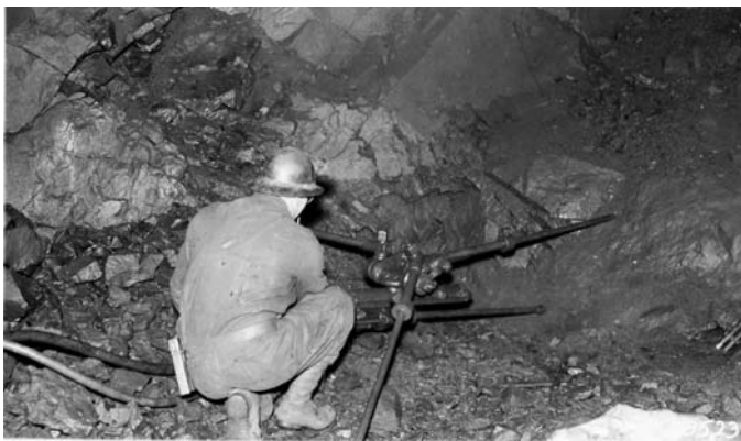
Figure 2. Wet drilling in an open stope with a Leyner Drill.
