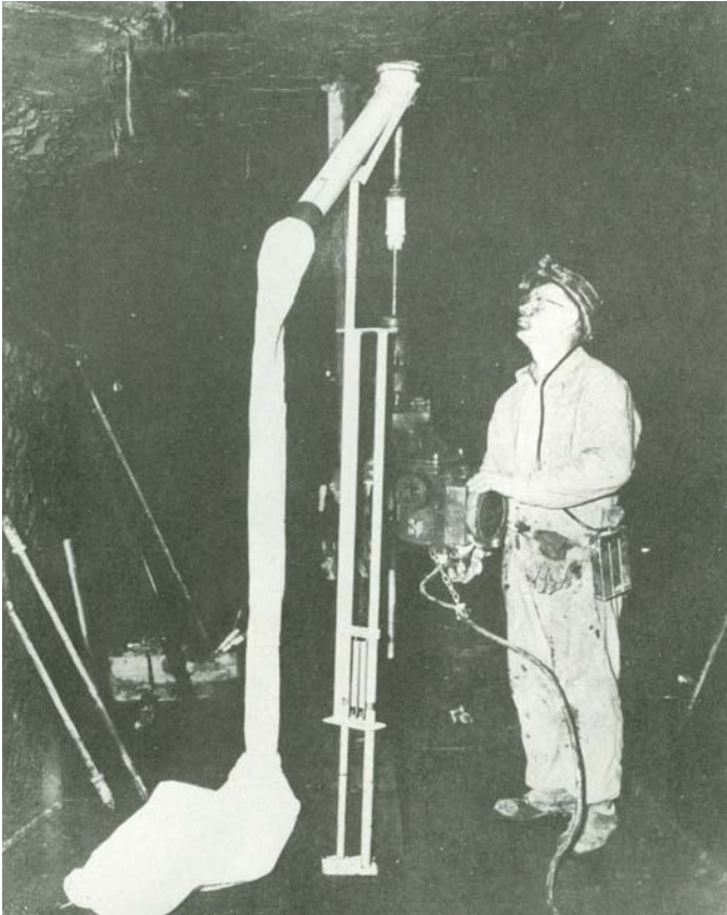
Figure 5. Testing a Browning dust collector.
