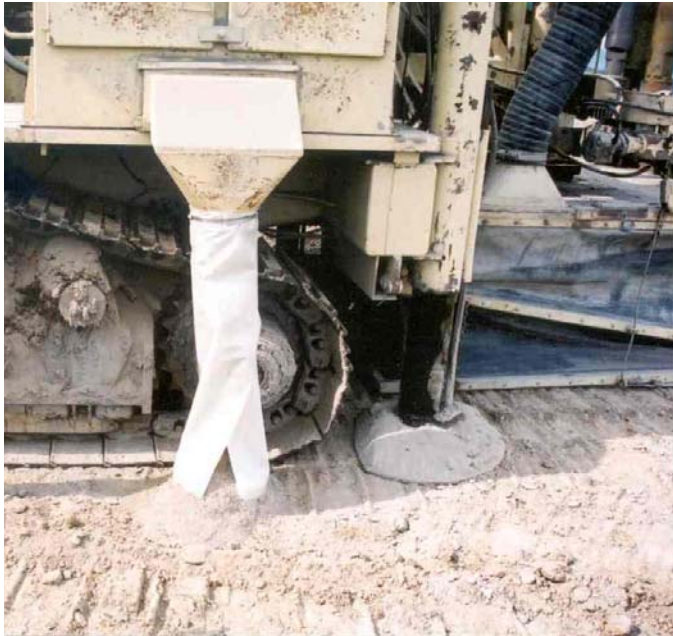
Figure 11. Dust collector dump point shroud.
