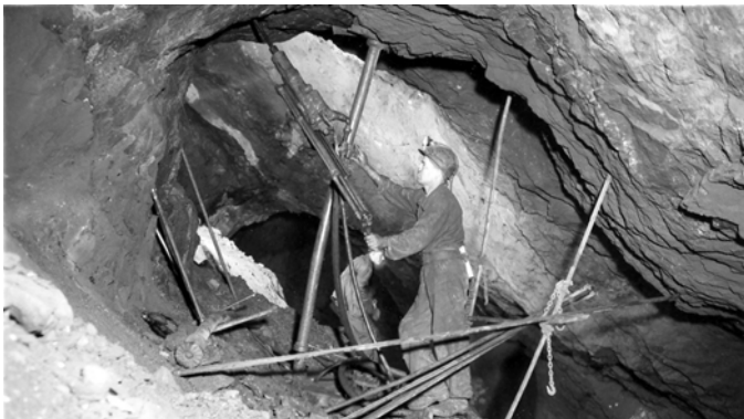
Figure 1. Angle drilling in an open stope.
