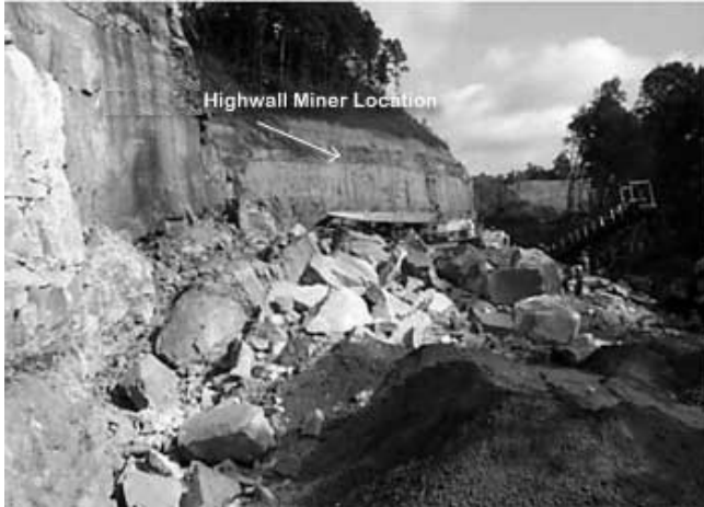
Figure 3 – Highwall collapse resulting in fatality
