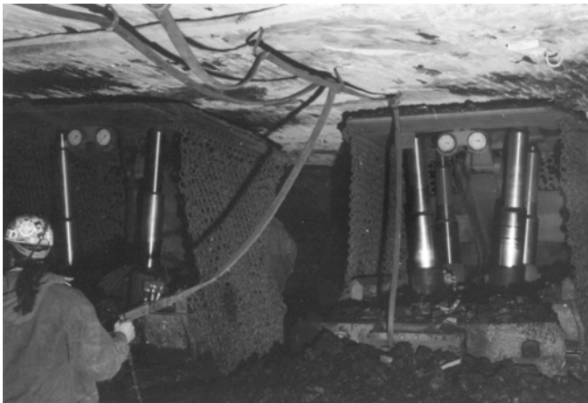
Figure 4. Full pillar extraction using mobile roof supports.
