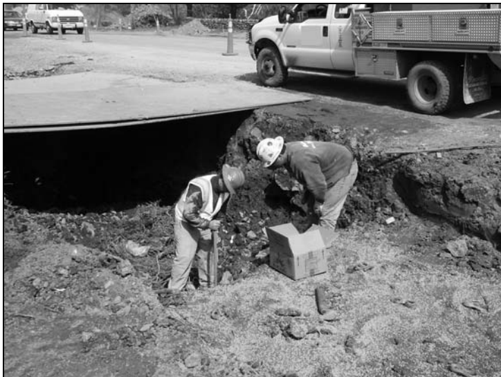
Figure 4 - Steel plates cover the open trench area.
