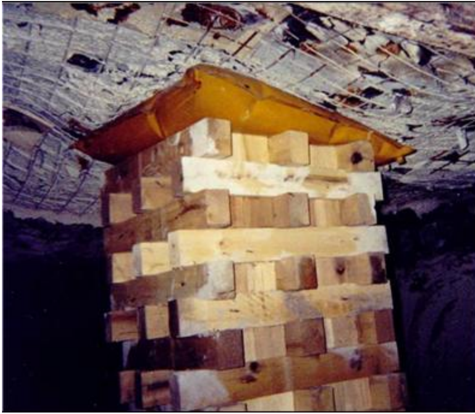
Figure 8: Application of prestressing bladder on a timber pack.
