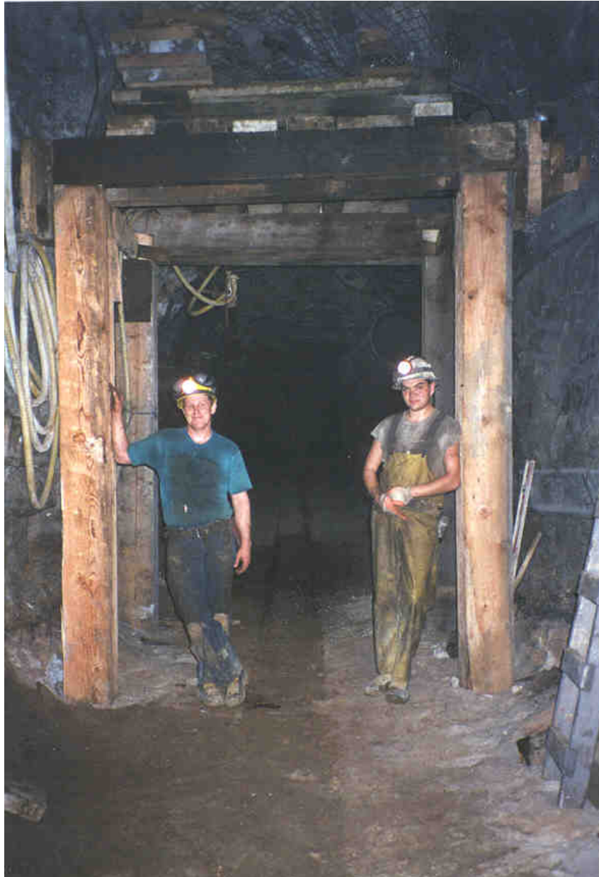
Figure 2: Traditional timber sets for hardrock applications.
