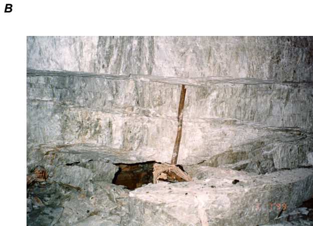
Figure 4. Cut (or drift) in a steeply dipping hard-rock vein. A, View along wall. Photo taken while standing on sandfill from previous cut. Note mining-induced fractures and temporary friction rock bolts from roof of previous cut exposed in wall. B, View of wall showing bent rock bolt offset by shear displacement along an echelon fracture zone.
