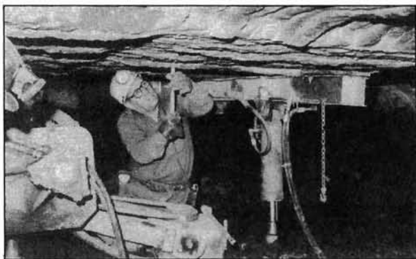
Figure 8.—Bolts installed in the mine roof help to prevent roof falls, thereby preventing fatalities and injuries to underground miners.
