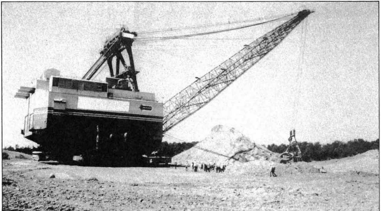
Figure 13.—Dragline used to remove overburden.
