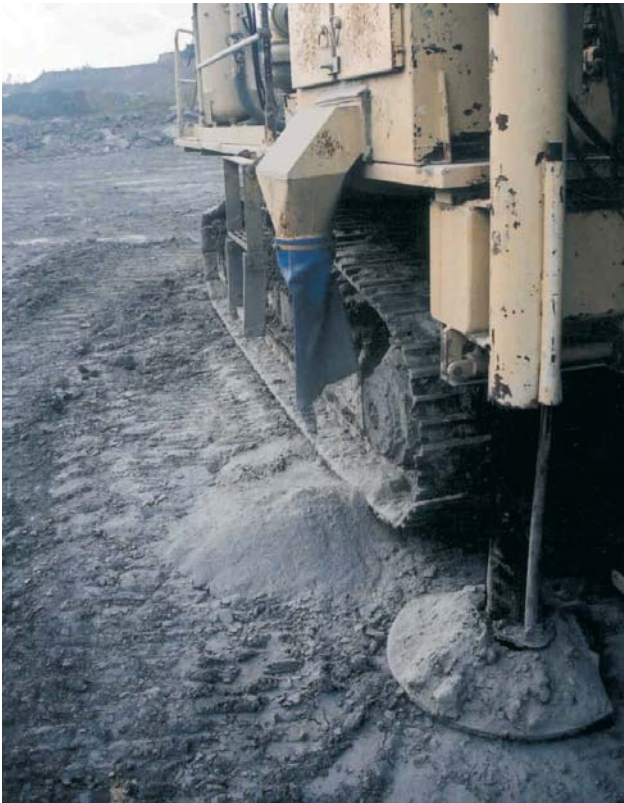
Dust collector dump point prior to installation.
