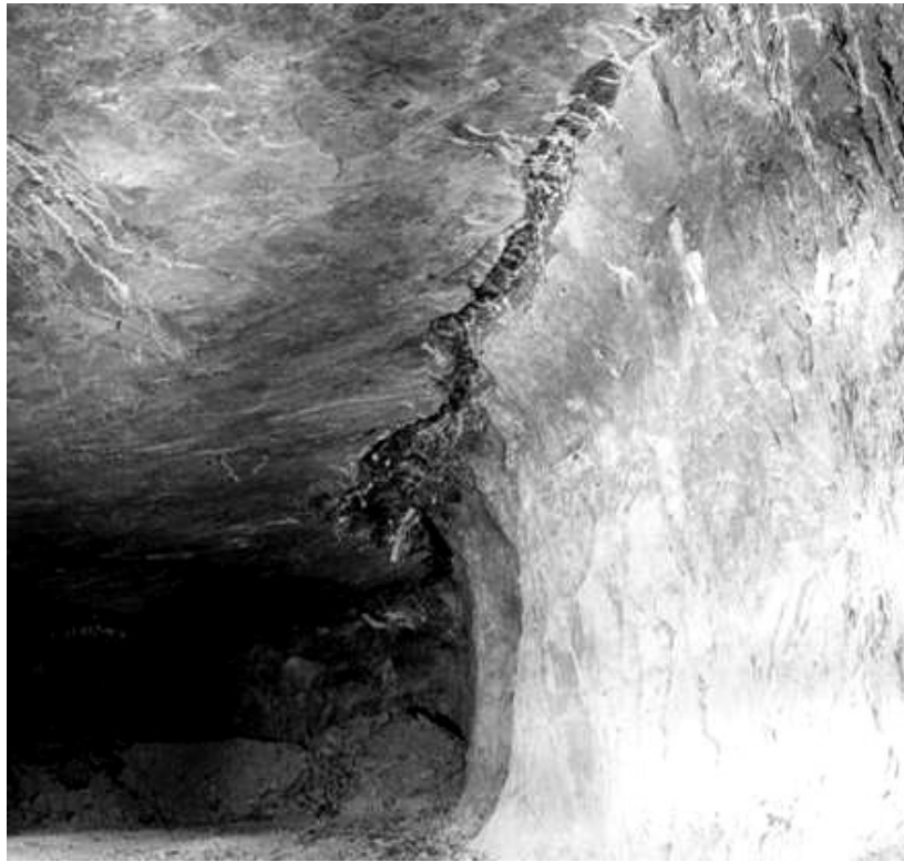
Figure 2. Roof guttering at the pillar-roof contact.
