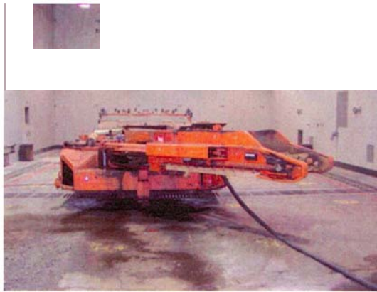
Illustration 4: The conveyor extended fully to the right.
