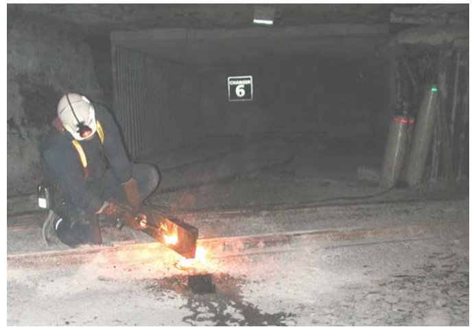
Figure 10. Flame cutting of a piece of rail.
