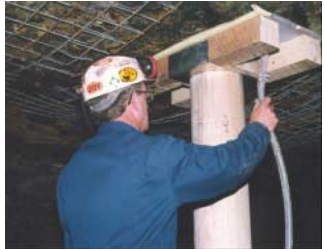
Figure 2. Propsetter grout bag has been the most commonly used prestressing system in the United States thus far.
