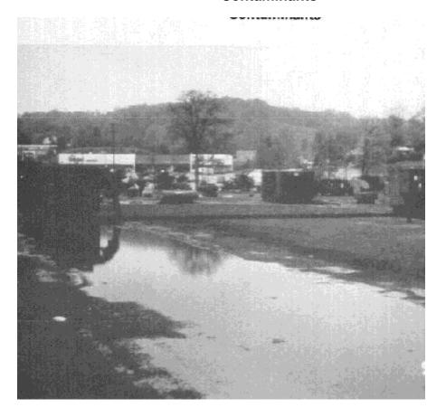
Standing water on a roof can cause water damage and potential mold growth sites inside the building as well as providing a breeding area for insects and microbiologicals such as Legionella. The outside air intake (near the far left of this photograph) is located close to the standing water and could be drawing in insects and microbiological contaminants.
