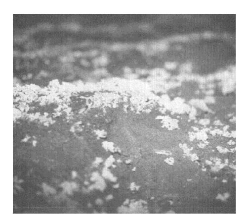
This is a school crawlspace in which moisture should be controlled. The fungus is Fusarium, some species of which are toxigenic and should not be inside. The spores were distributed by the air handler because the return plenum was open to the crawlspace.
