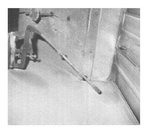
Malfunctioning controls such as this broken damper linkage can virtually eliminate intake of outdoor air. Such problems may go undetected for years without a careful investigation of the HVAC system components.
