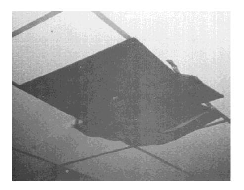
Complaining of discomfort, building occupants blocked air supply diffusers in their work areas. The HVAC system in this building was in poor condition and was not balanced.
