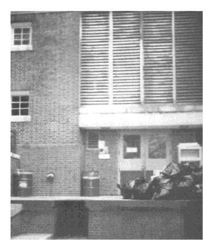
Air intakes are frequently located near the loading dock for aesthetic reasons. Unfortunately, this air intake placement can draw car and truck exhaust into the building, causing a variety of indoor air quality complaints.
