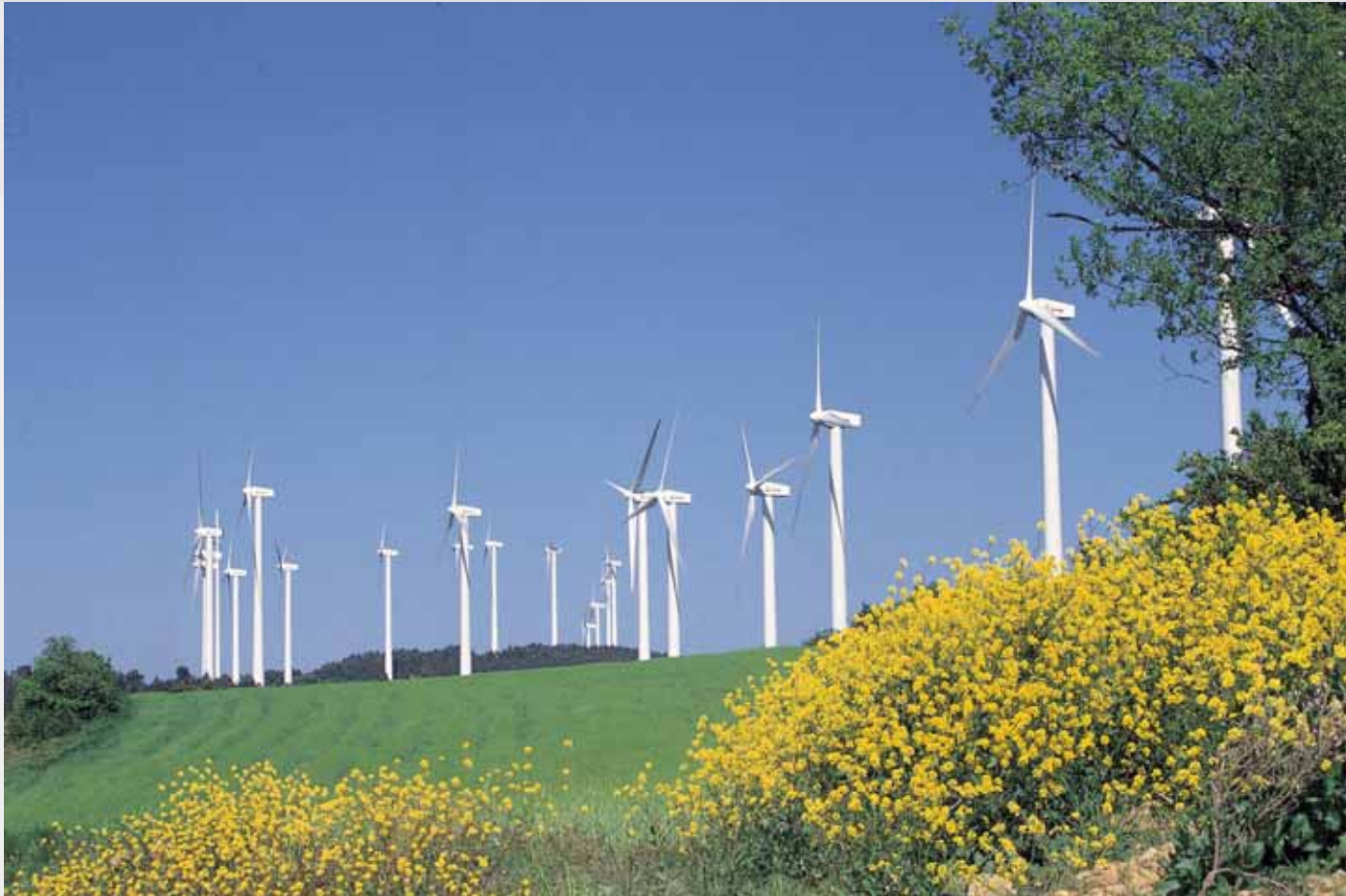
Windpark in the Izco range of hills (Navarre, Spain)
