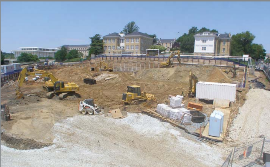
Construction Site, May 15, 2008
