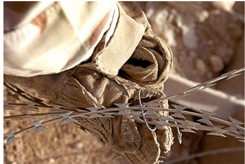
U.S. Air Force Senior Airman Margaret Wilson connects two lengths of concertina wire together, on a wall to protect one of the compounds on Ali Air Base, Iraq. Wilson is assigned to the 407th Expeditionary Security Forces Squadron's Force Protection Flight. The flight is responsible for monitoring local and third country nationals to detect suspicious activity, augmenting security forces during increased threat levels, as well as monitoring and maintaining installation security measures.
