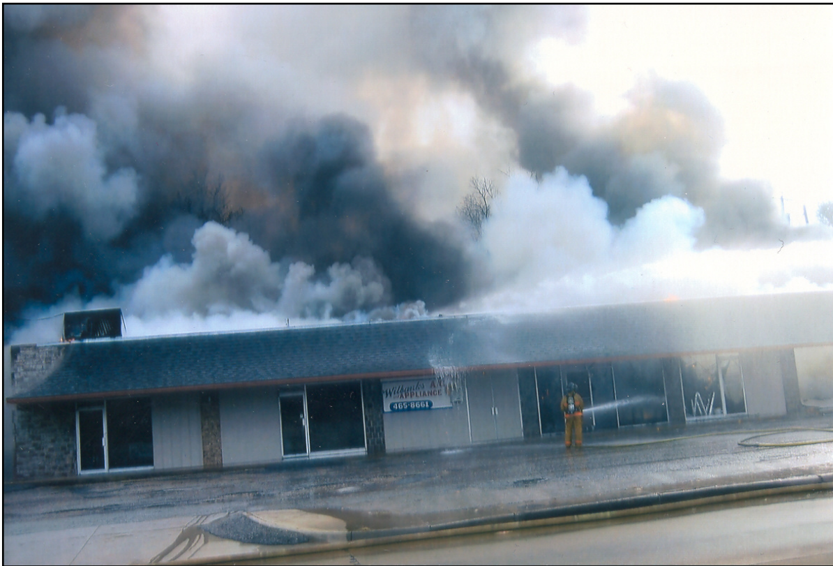
Photo 1. Front of incident structure prior to awning collapse. Photo courtesy of fire department.
