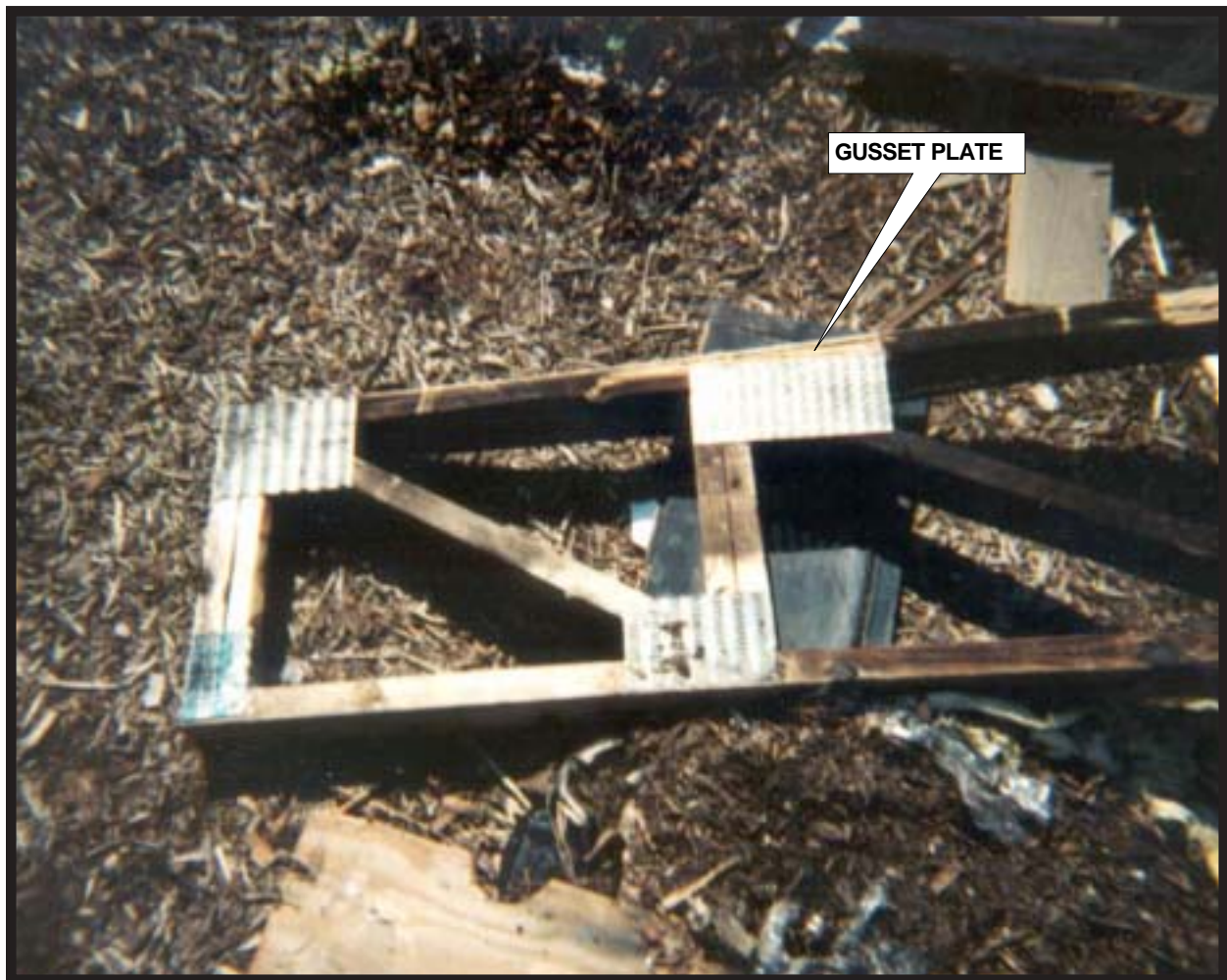
Photo 2. Lightweight wooden parallel-chord truss
