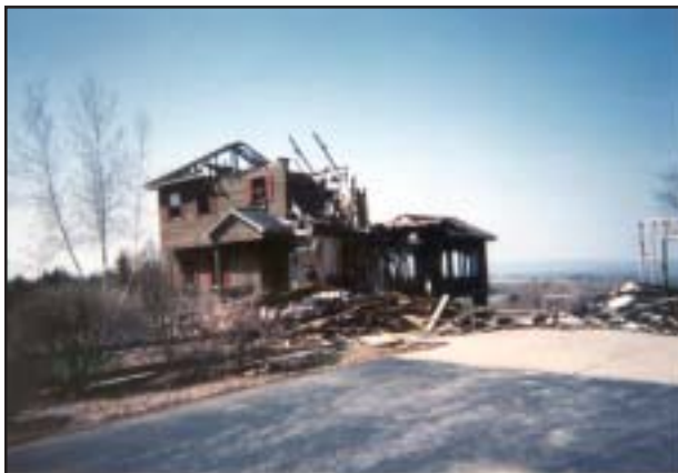
Front of Structure
