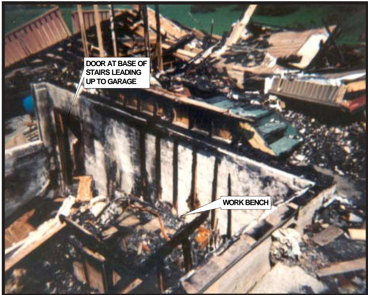
Photo 1: Basement area into which victims fell
