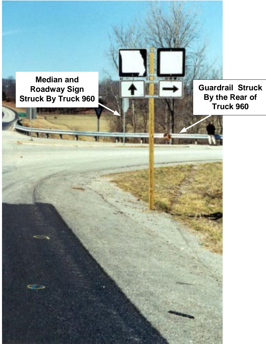
Photo 1. Median and Guardrail Struck By Truck 960
