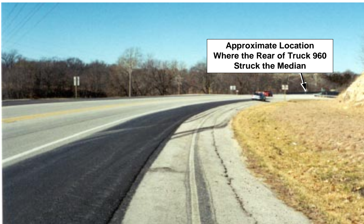
Photo 2. The Curve on the Road Where the Victim was Traveling
