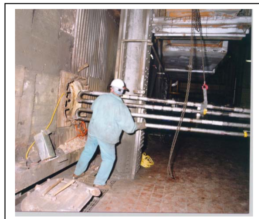
Figure 5: Installation into Niles Boiler
