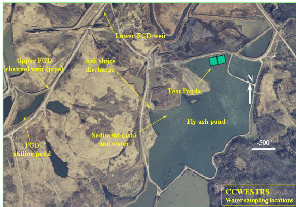
Fig. 1. Aerial photograph showing fly ash ponds and test ponds at Paradise Power Plant.
