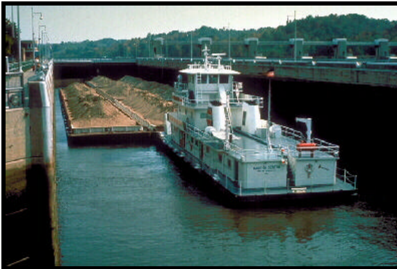
A tow enters the chamber at Cheatham Lock.
